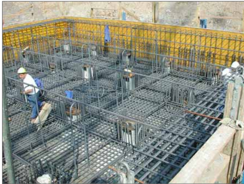
Injected piles for bridge pier foundations Viaduct at José (B)
