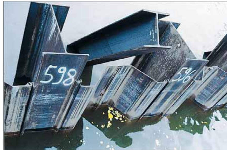
Raked steel piles working in tension
