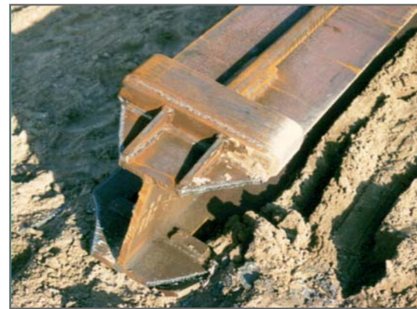
Toes of HP-injection piles 32
