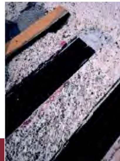
Lamine prefabbricate poste in opera
