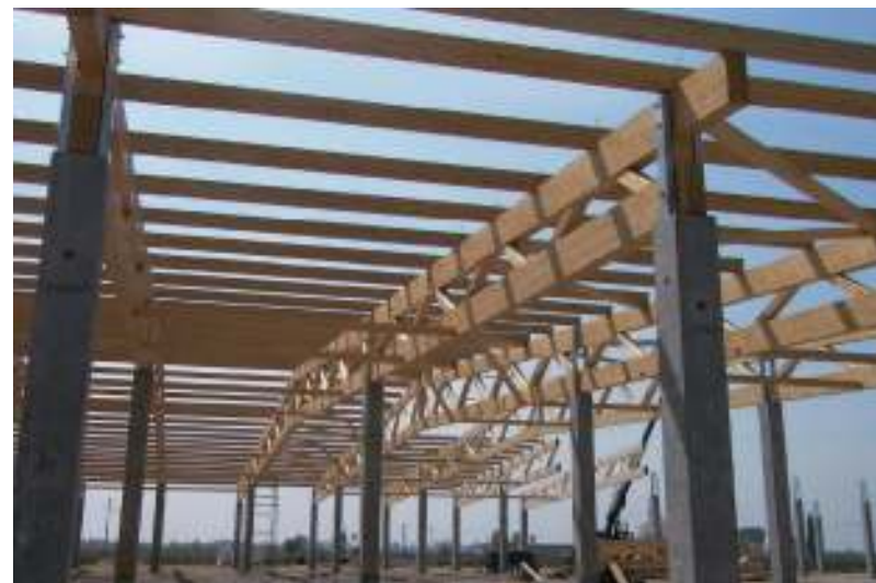
Pilastro in c.a.
